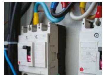
CIRCUIT BREAKER VAMPGREEN Y 30G RC V0 28 HF 1S 04 PA66, 30% glass fibre reinforced, UL 94 V0 halogen free
