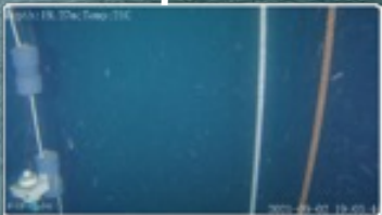
Internal Pile Inspections
