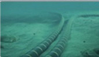
Submarine Cable Maintenance
