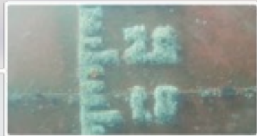
Ballast Gauge Inspections
