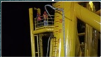
Jacket Grout Inspections
