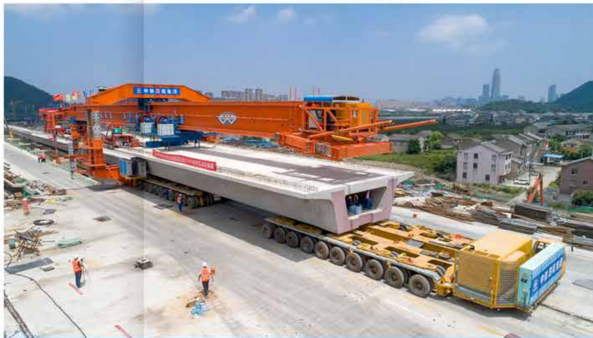
DELIVERY THE GIRDER FOR BEAM ERECTOR
