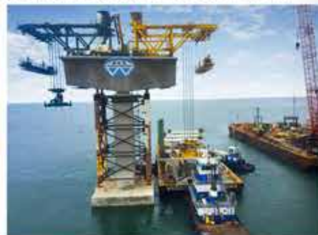
▶ SE120 IN MARC BASNIGHT BRIDGE PROJECT, USA
