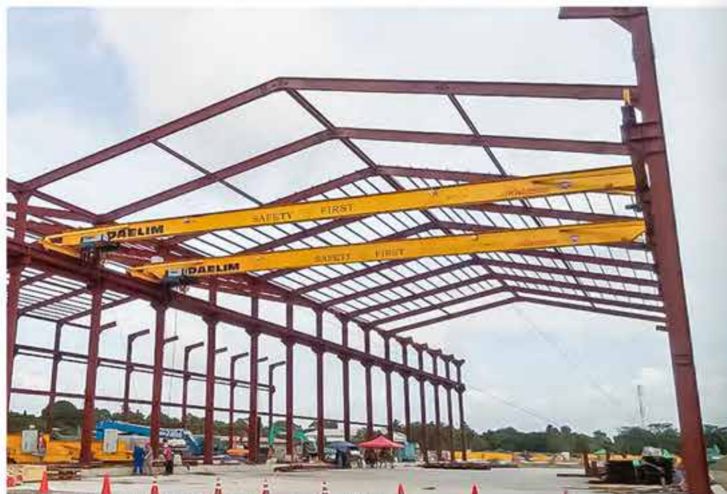
▶ OVERHEAD CRANE IN TEMBURONG BRIDGE PROJECT, BRUNEI
