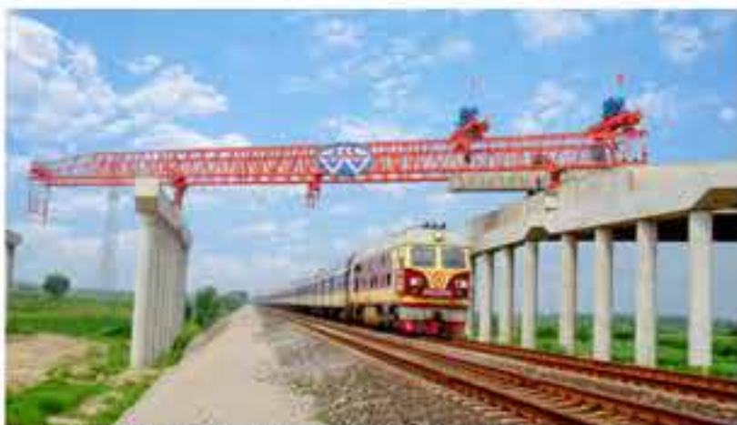
▶ DJ40200 IN CROSS EXISTING LINES PROJECT, CHINA
