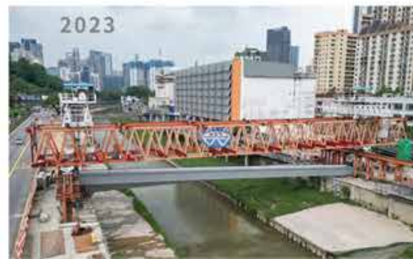
▶ JSHB67220 IN BRICKFIELD BRIDGE PROJECT, MALAYSIA
