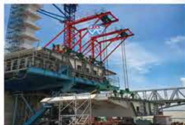
▶ SE120 IN BAGO BRIDGE PROJECT, MYANMAR
