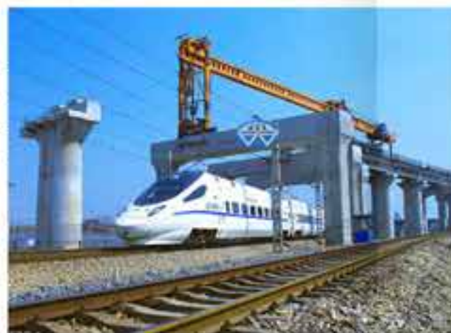
▶ DJ40180 IN RAILWAY PROJECT, CHINA
