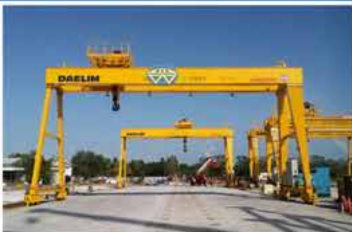
▶ QLH80 IN TEMBURONG BRIDGE PROJECT, BRUNEI
