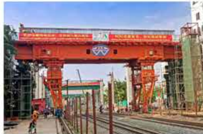
▶ HMQ60 IN DHAKA AIRPORT PROJECT, BANGLADESH
