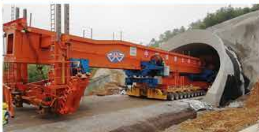
DELIVERY THE BEAM ERECTOR THROUGH TUNNEL
