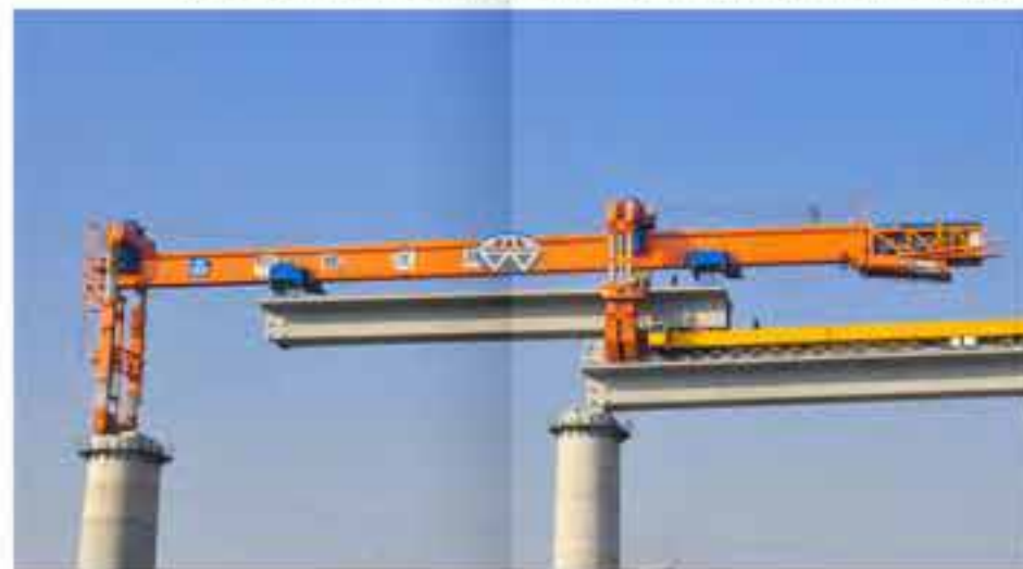
▶ DJ600 IN QINGDAO-JINAN HIGH-SPEED RAILWAY PROJECT, CHINA
