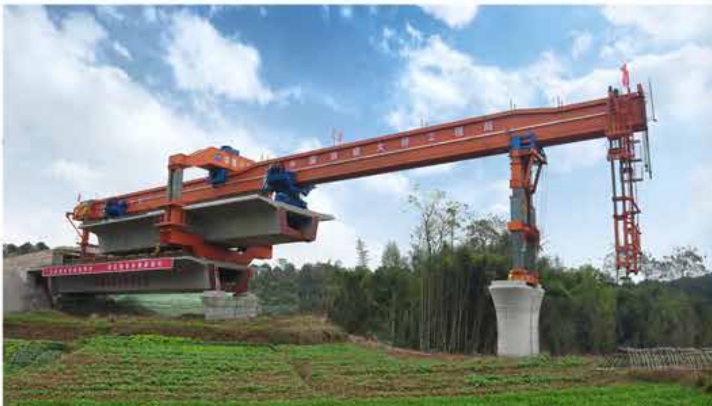
HANGSHAOTAI HIGH-SPEED RAILWAY PROJECT (CRCC), CHINA
