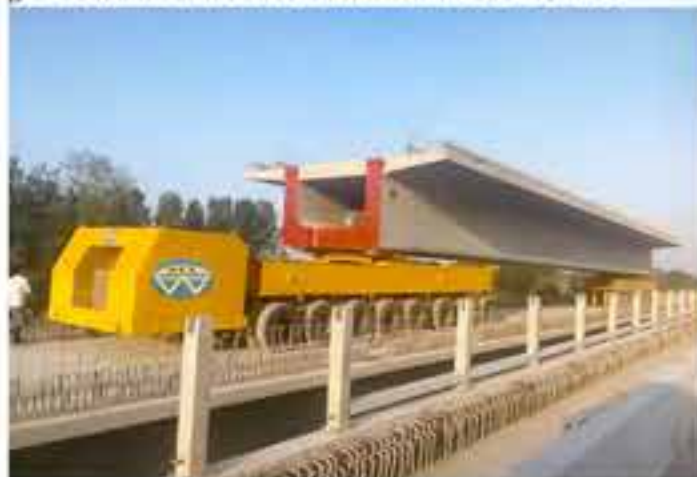
► YLC600 IN JIQING HIGH-SPEED RAILWAY PROJECT, CHINA
