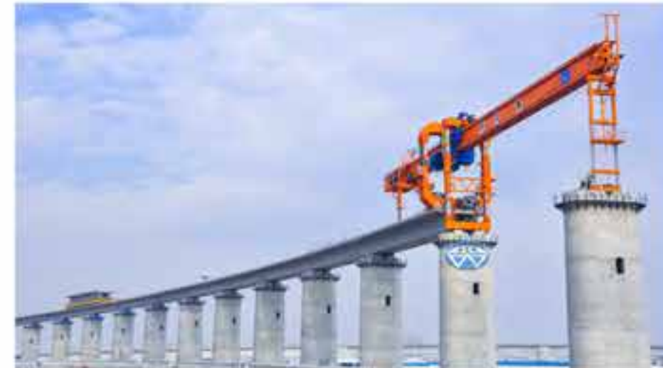
▶ DJ600 IN XUZHOU-YANCHENG HIGH-SPEED RAILWAY PROJECT, CHINA
