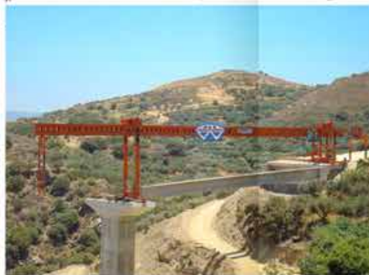
▶ DJ40100 IN METSOVITIKOS BRIDGE PROJECT, GREECE
