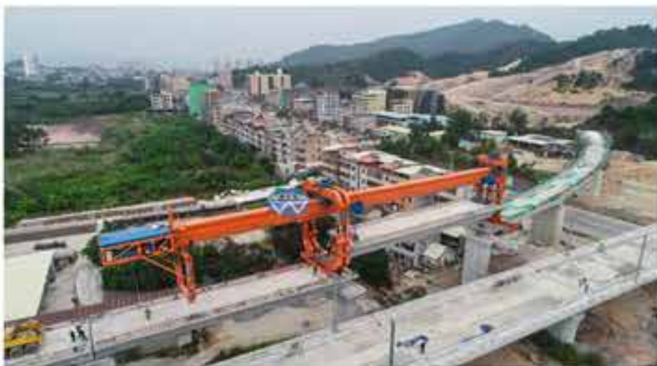
▶ DJ550 IN GANZHOU-SHENZHEN HIGH-SPEED RAILWAY PROJECT, CHINA
