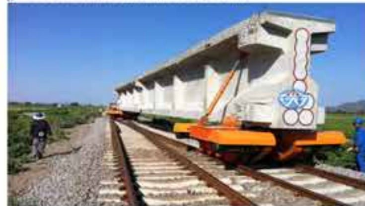
► TYLC180 IN RAILWAY PROJECT, CHINA
