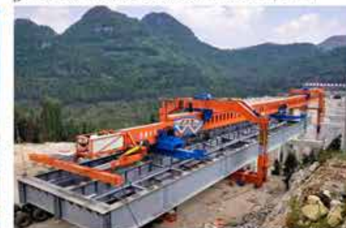
▶ DJ48220 IN STEEL BOX GIRDER PROJECT, CHINA
