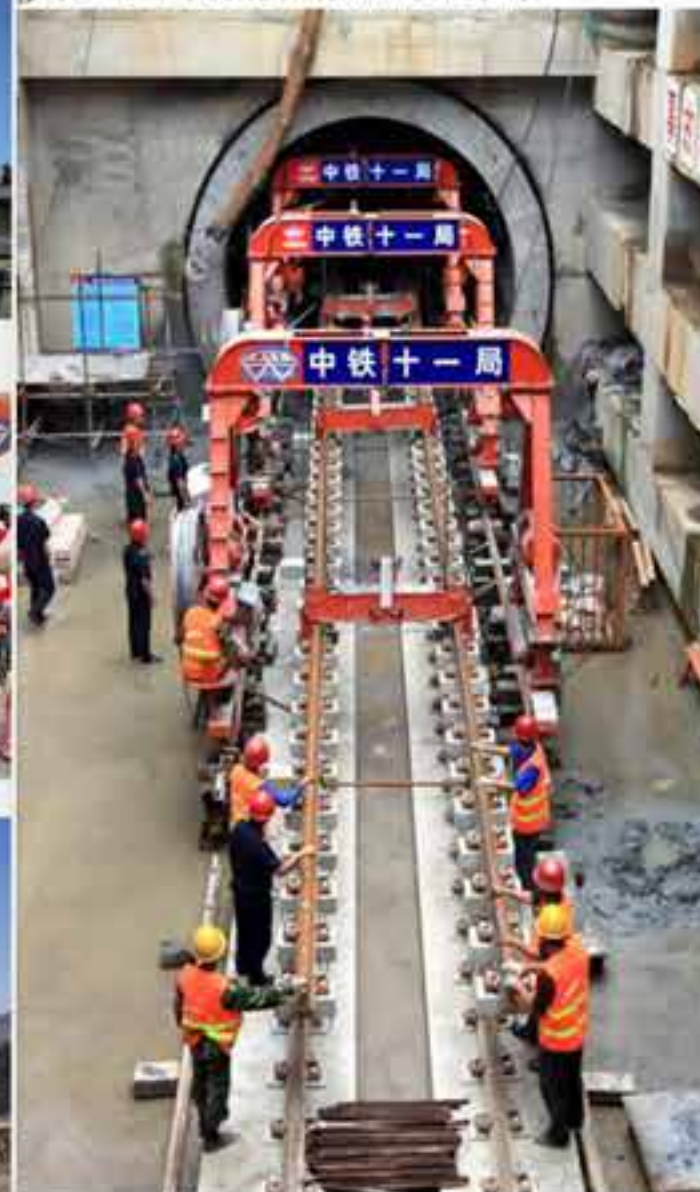
> METRO ENTRANCE CONSTRUCTION
