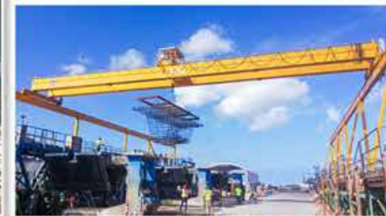
▶ OVERHEAD CRANE IN HONOLULU RAIL TRANSIT PROJECT, USA
