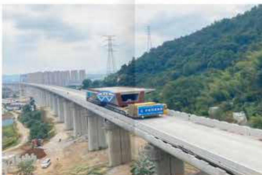
DELIVERY THE GIRDER ON THE BRIDGE
