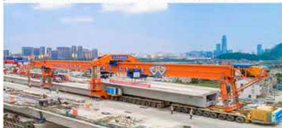
HANGSHAOTAI HIGH-SPEED RAILWAY PROJECT (CREC), CHINA
