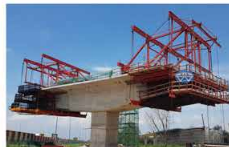
▶ FT150 IN GAMUDA COVE BRIDGE PROJECT, MALAYSIA
