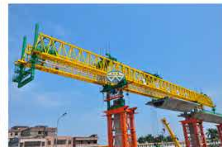
▶ LG40 IN GUANGZHOU METRO LINE 14 PROJECT, CHINA
