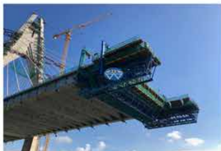
▶ FT630 IN TEMBURONG BRIDGE PROJECT, BRUNEI
