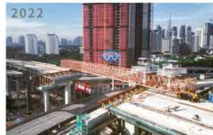
▶ JSHB67220 IN MAINLINE DUKE 3 PROJECT, MALAYSIA
