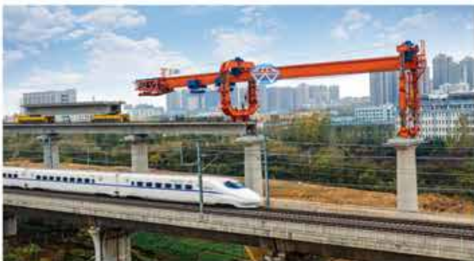
▶ DJ550 IN HEFEI-ANQING HIGH-SPEED RAILWAY PROJECT, CHINA
