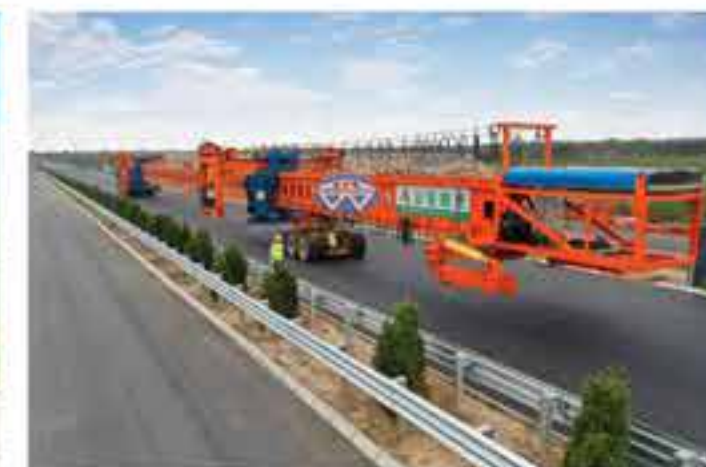
▶ DJ40180 IN BINBO EXPRESSWAY PROJECT, CHINA
