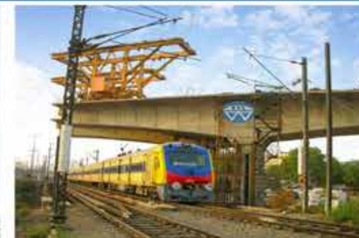
▶ SE300 IN BARAPULLA ELEVATED HIGHWAY, INDIA
