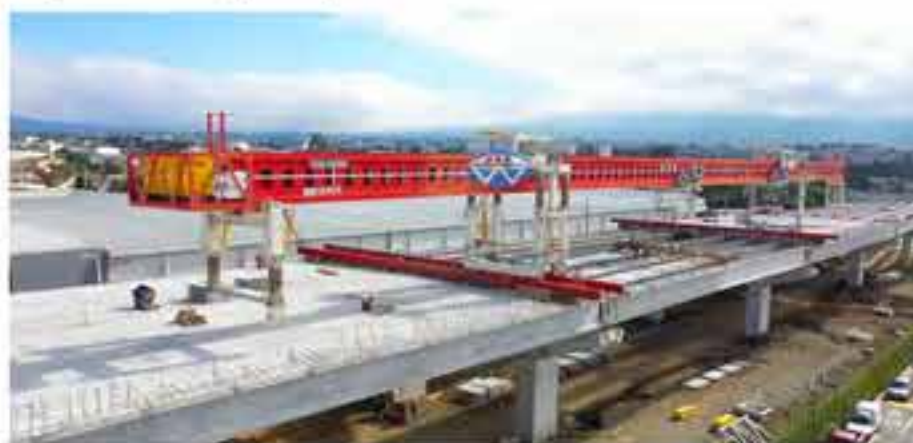
▶ DJ50160 IN SAN JOSE NORTH RING ROAD PROJECT, COSTA RICA
