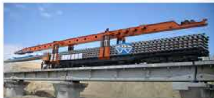
> DJ32 TRACK LAYER IN CHINA PROJECT
