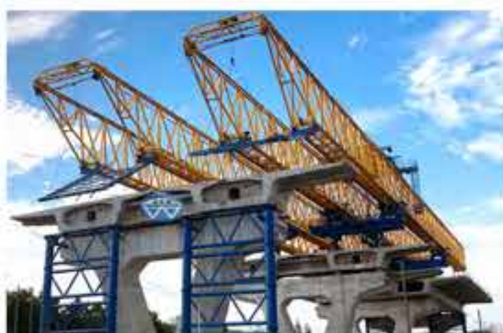
▶ LG80/100 IN HANGSHAOTAI PROJECT, CHINA
