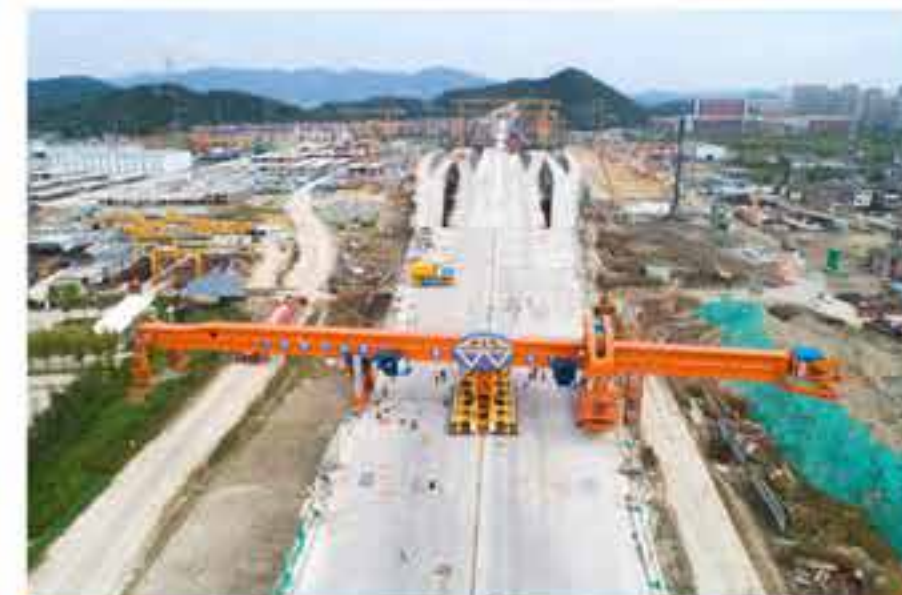
ASSIST BEAM ERECTOR TO TURN AROUND
