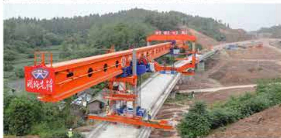
SHANGHAI-CHONGQING-CHENGDU HIGH-SPEED RAILWAY PROJECT, CHINA
