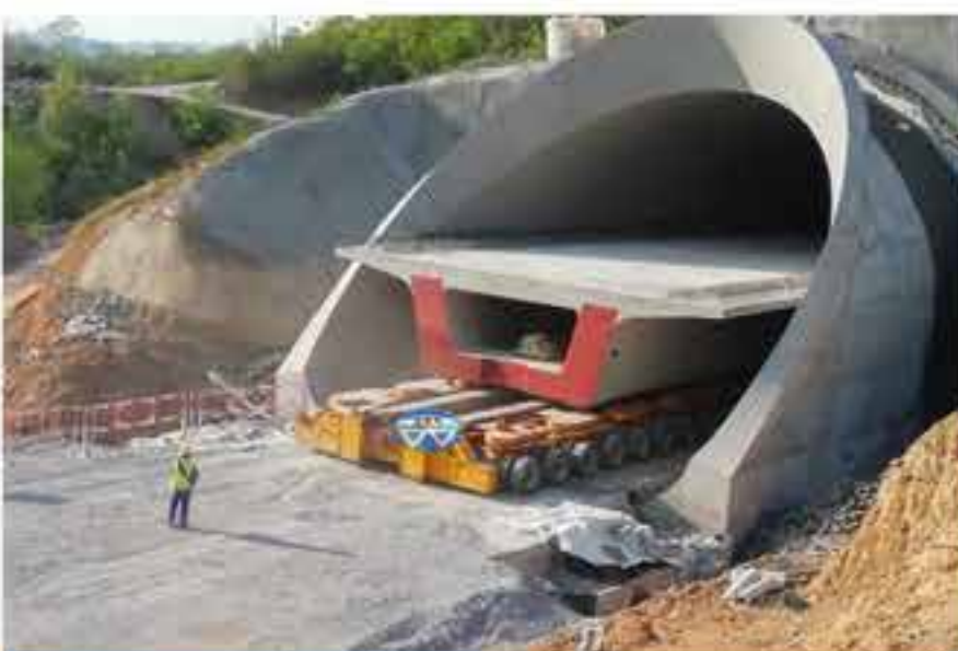
DELIVERY THE GIRDER THROUGH THE TUNNEL
