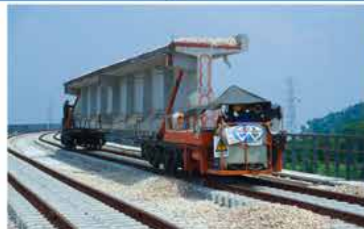
► TYLC180 IN RAILWAY PROJECT, CHINA
