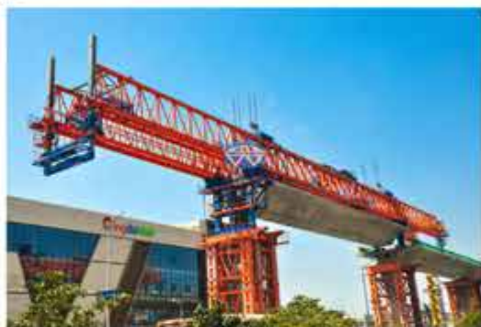
▶ LG60 IN GUANGZHOU METRO LINE 14 PROJECT, CHINA
