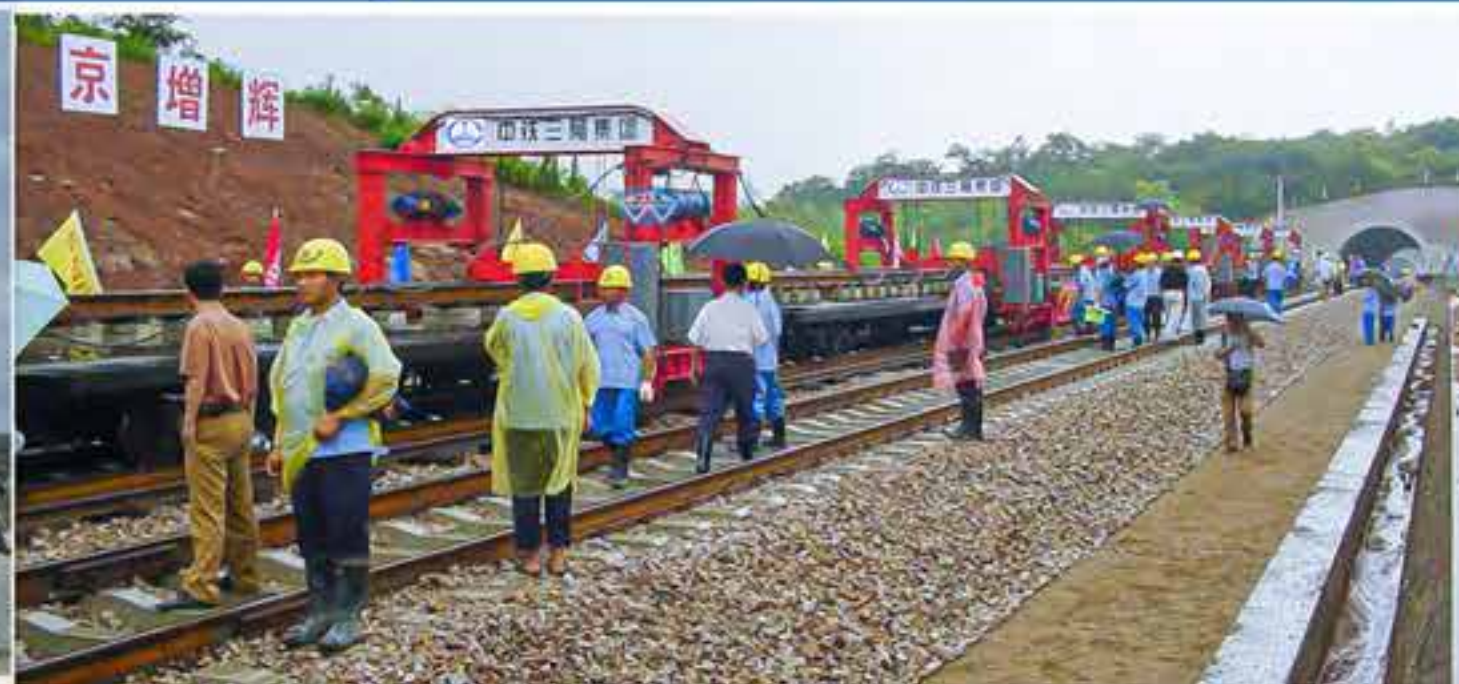
> 125 METERS LONG TRACK CONSTRUCTION
