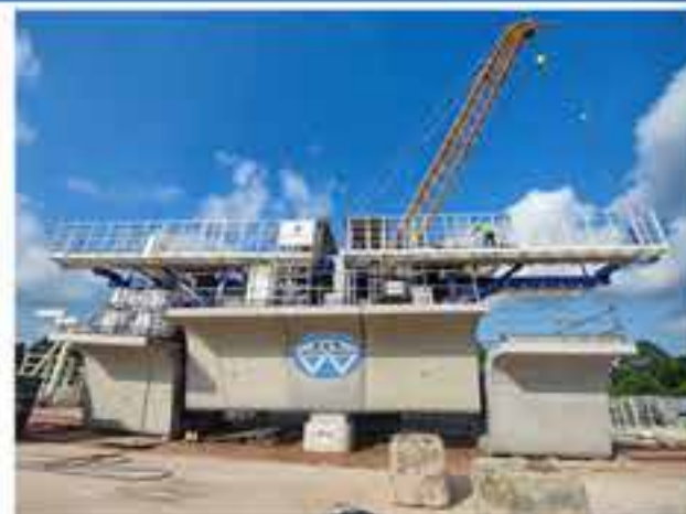
▶ SE65 IN JURONG-LINE ITTC PROJECT, SINGAPORE
