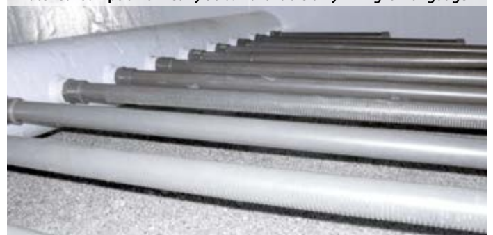
► Refurbishment of swimming pool filter achieves a reduction of fresh water consumption of nearly 50 % – available only in English language
