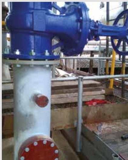
New valve installed
