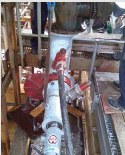
Old valve removal
