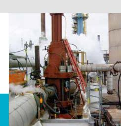
The design of the blind plate and the pipe holding assembly allows the pipe to be temporarily closed for several days, months and even years until the next planned shutdown of the technological process, or repeated commissioning, after the defect or problem has been rectified.
