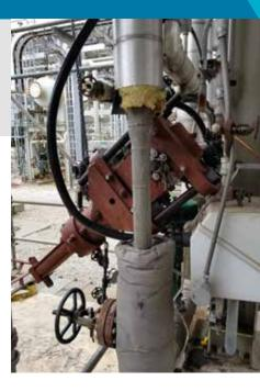
PLIDCO® SHEAR+PLUG isolating technology is used on the in-service piping containing gaseous or liquid products from DN20 (3/4") to DN450 (18"). This maintains the maximum productivity of the piping system even during the repair works, as there is no need to interrupt or shutdown the technological processes, thereby reducing the financial losses caused by a possible shutdown.
