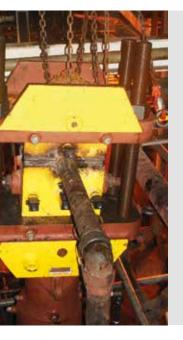
A pipe holding assembly is welded on the in-service pipe. The hydraulic device with a shear blade is installed on the pipe holding assembly and then, without a need for piping shutdown, it cuts the pipe and closes the pipe at the cut-off point. A coupon is caught in the coupon receptacle housing and then removed.
