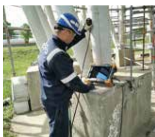
Corrosion under fireproofing (CUF)
