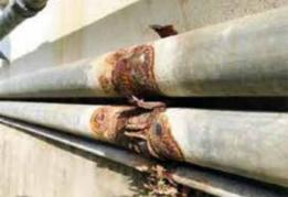
The method of Pulsed Eddy Current Array measuring (PECA<sup>™</sup> or PEC), is an advanced electromagnetic NDT technology ideal for quick detection of material losses (corrosion) especially under insulation (coating) or fireproofing.
